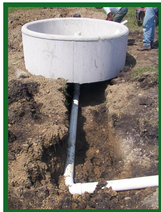
Bury permanent piping underground.
