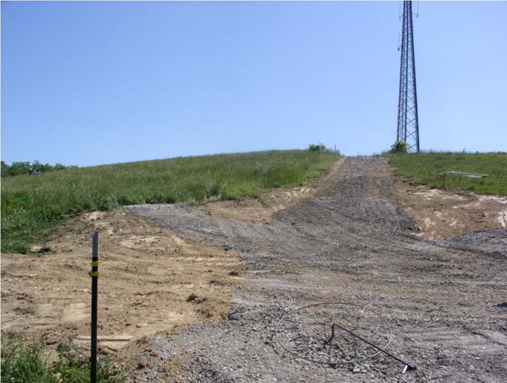
Alleyway stabilization, Westmoreland County.
