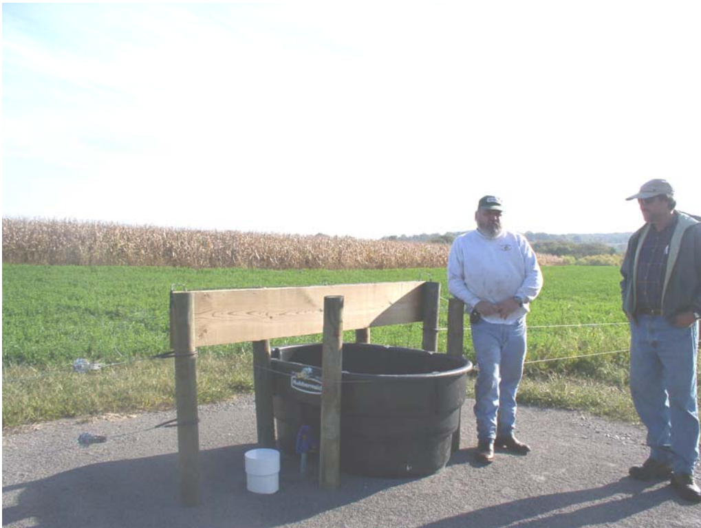
Watering facility Armstrong County.
