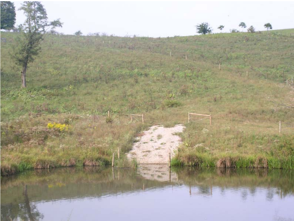
Pond access ramp and stream buffer Fayette County.
